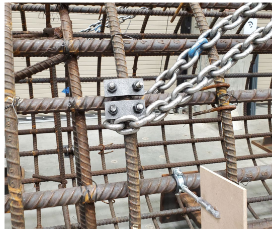
Fig. 9. Pick-up points at the intersection of tied-hoops and pick-up bars
