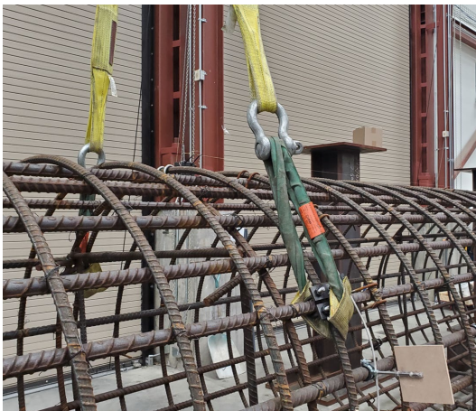
Fig. 9. Pick-up points at the intersection of tied-hoops and pick-up bars
