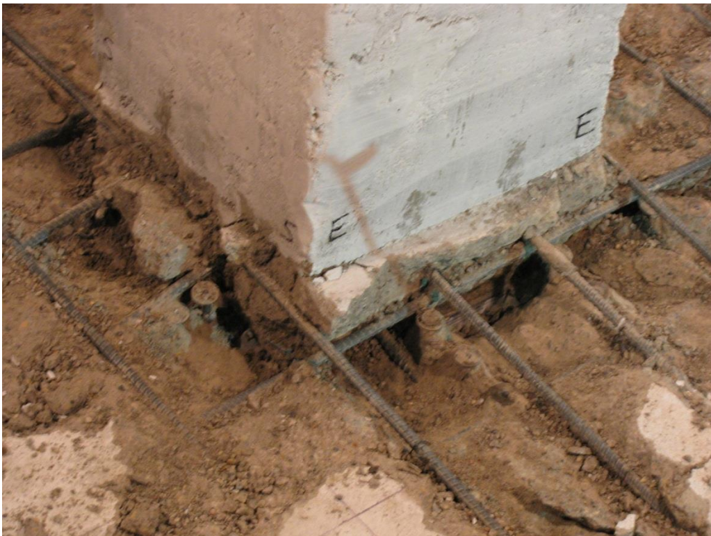
Figure 4-24: Specimen B3 – Void in Connection Region after Loose Concrete was Removed
