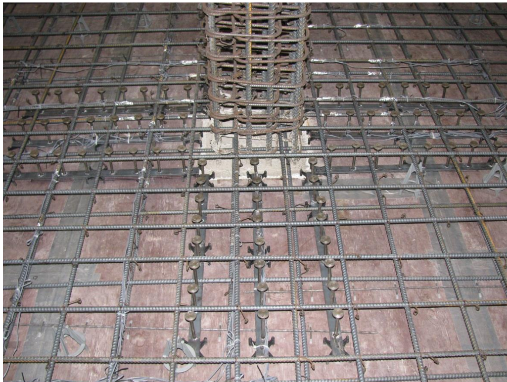
Figure 1-2: Orthogonal Stud Rail Arrangement
