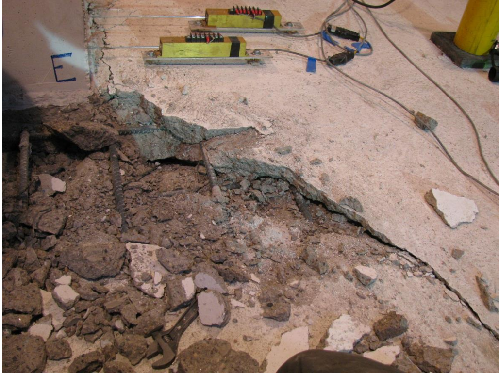
Figure 3-3: Specimen B1 – Diagonal, Radial Crack at Northeast Column Corner
