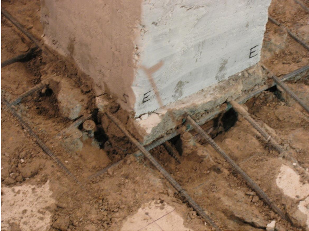
Figure 3-18: Specimen B3 – Void in Connection Region after Loose Concrete was Removed After Test
