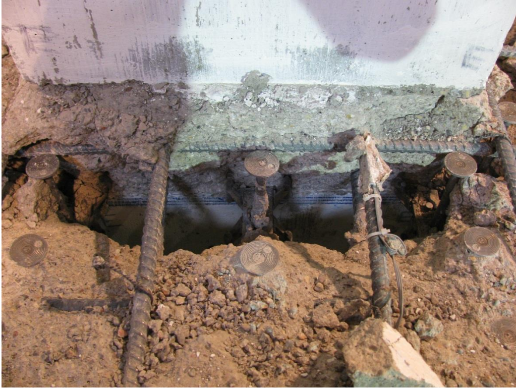
Figure 4-23: Specimen B2 – Connection Region where Damaged Concrete was Removed by Hand
