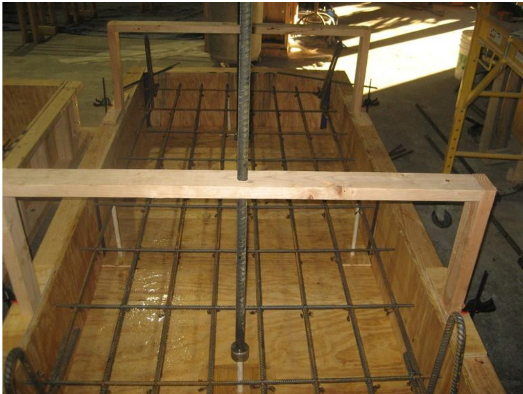
Figure 2.29 Shallow embedment specimen formwork
