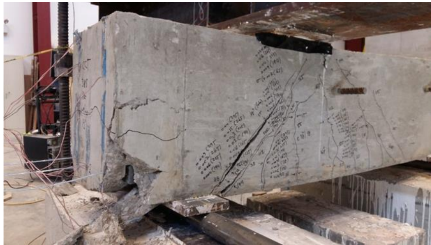
Figure 4.2 Specimen H-3-8-5-13-F4.1-II after failure
