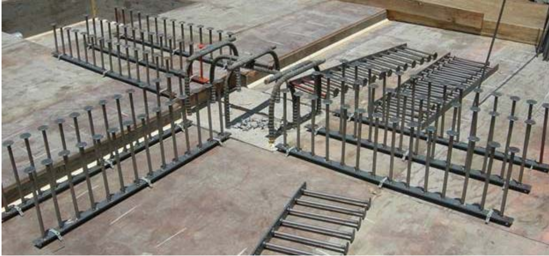
Figure 1.9: Stud rails used to increase the punching shear resistance of reinforced concrete slabs
