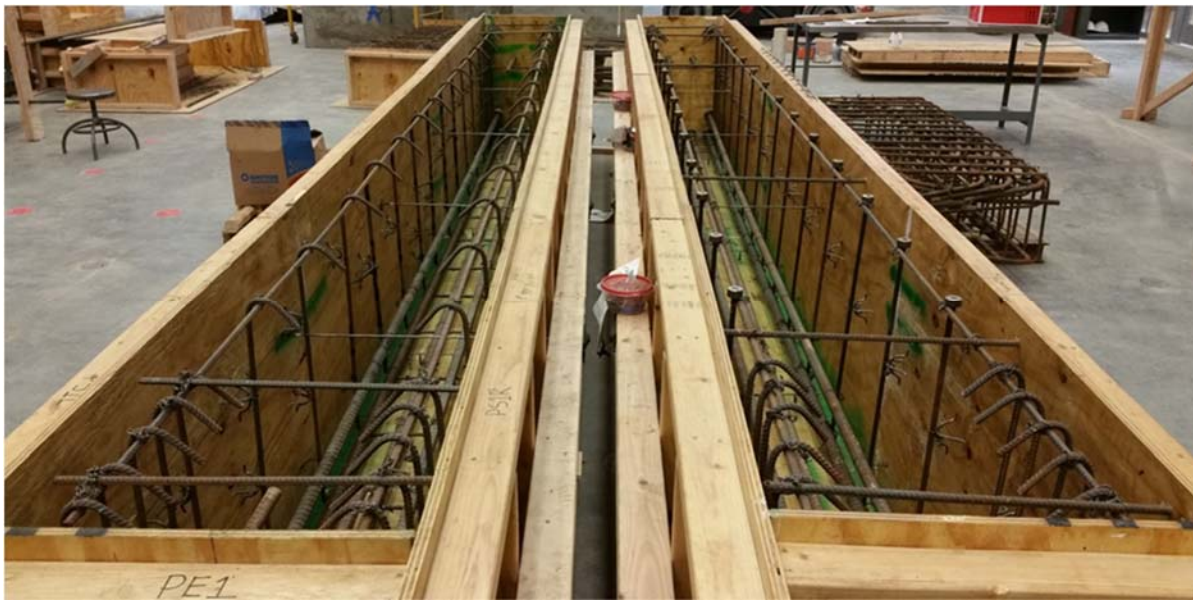
Figure 2.4: Reinforcement cages with conventional stirrups (left) and headed bars (right) as shear reinforcement
