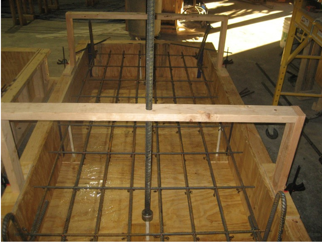
Figure 2.6 Slab specimen formwork
