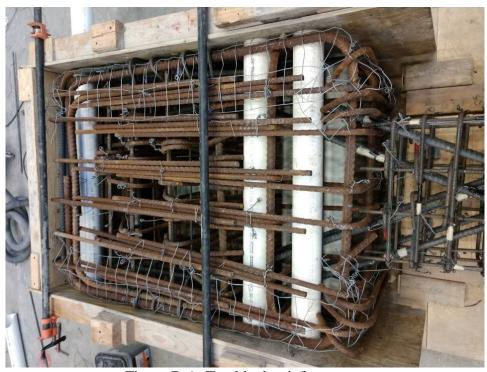
Figure B.6 –Top block reinforcement typical of beams with aspect ratios of 2.5 and 3.5
