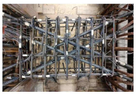
Figure B.1 – Coupling beam reinforcement, D120-1.5
