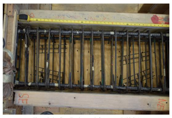
Figure B.4 – Coupling beam reinforcement, P100-2.5
