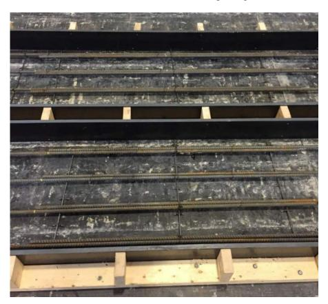
Figure 3.13: Slab Construction – Splice Region
