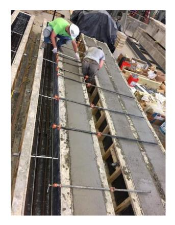
Figure 4.23: Series VI Form Bracing
