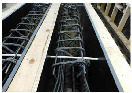
Figure 2.17: Reinforcing Cages Inside Forms
