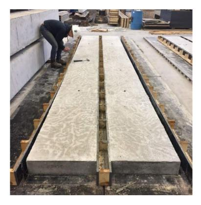
Figure 3.20: Series V Side Form Removal
