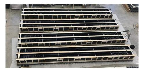
Figure 2.16: Completed Formwork
