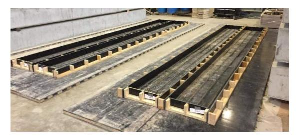
Figure 3.11: Series V Completed Formwork
