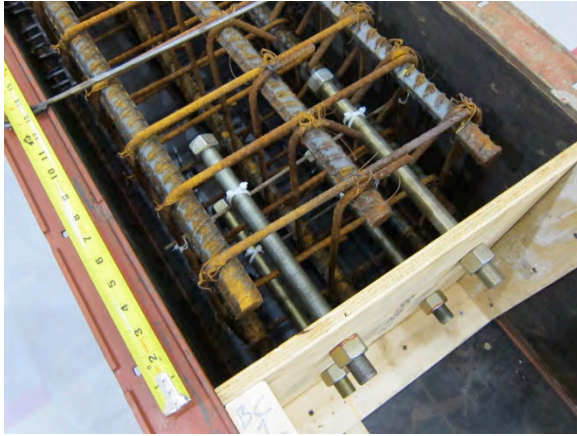
Detail of hinge assembly at the top and bottom of the column
