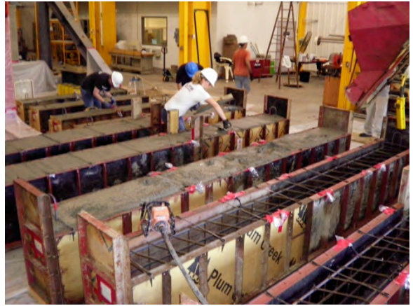
Figure C.3: Formwork
