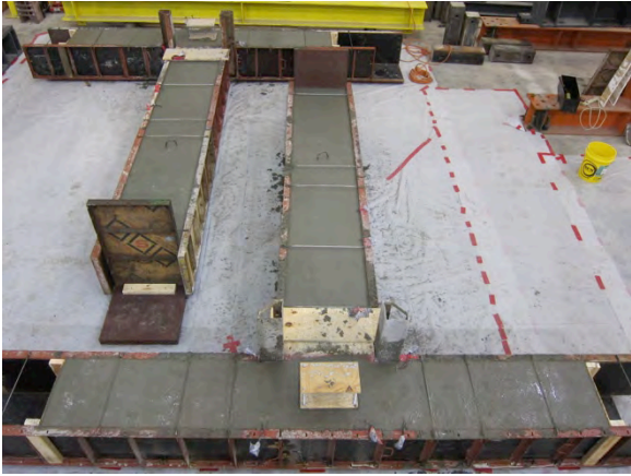
After placement of concrete
