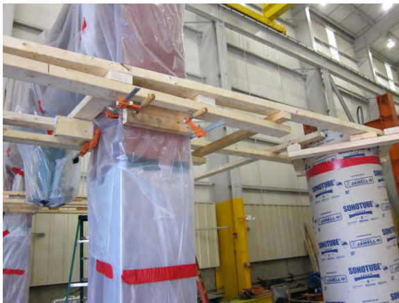
Figure H.2: Formwork
