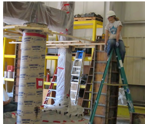
Figure H.2: Formwork
