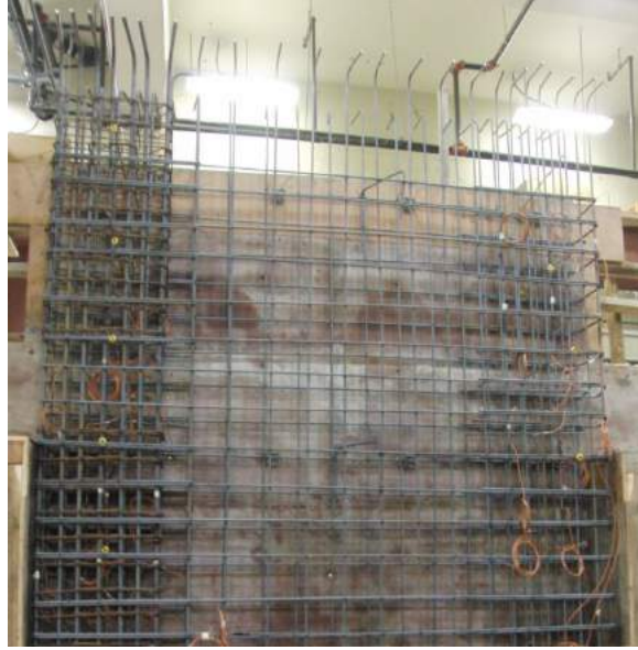
Figure 4.3: Structural Wall Reinforcement for Sub-Assembly #2 (with SRC3 and SRC4)
