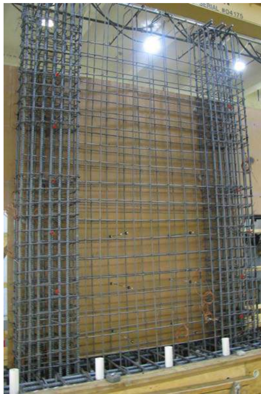
Figure 4.2: Structural Wall Reinforcement for Sub-Assembly #1 (with SRC1 and SRC2)
