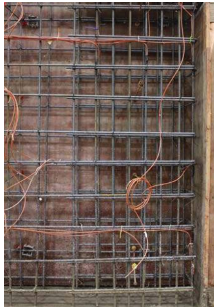
Figure 4.10: No Wall Boundary Transverse Reinforcement
