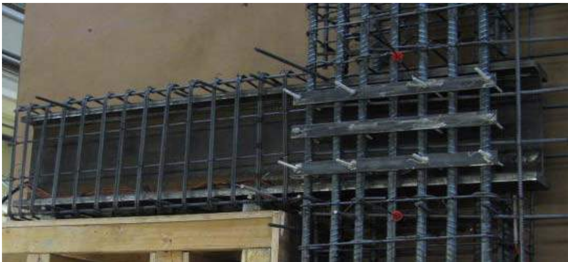
Figure 4.6: SRC2 Embedded Steel Section and Reinforcement
