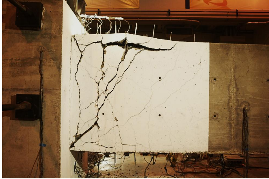
Figure 10 Beam 1: buckling of the top longitudinal bars (first cycle with peak drift ratio = 2.7%, instantaneous drift ratio = 2.7%).
