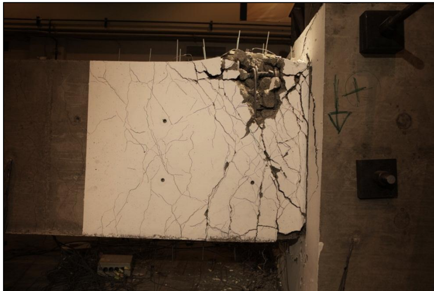
Figure 26 Beam 2: damage state at the beginning of the displacement cycle in which bottom longitudinal reinforcement buckled (maximum drift ratio = 5.3 %, instantaneous drift ratio = 0.8%).
