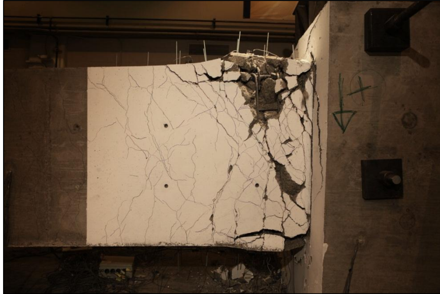
Figure 27 Beam 2: buckling of bottom longitudinal reinforcement (instantaneous drift ratio equal to peak cycle drift ratio of 5.3%).
