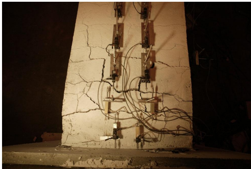
Figure 24 Beam 2: top view of damage state (first cycle with peak drift ratio = 2.9%, instantaneous drift ratio = -2.9%).
