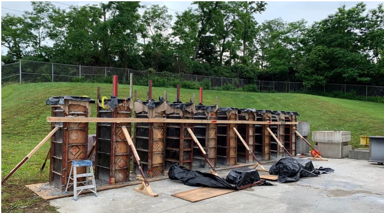
Figure 2.6 Formwork and curing
