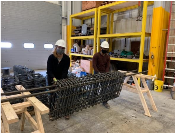
(a) Tying of reinforcement cages
