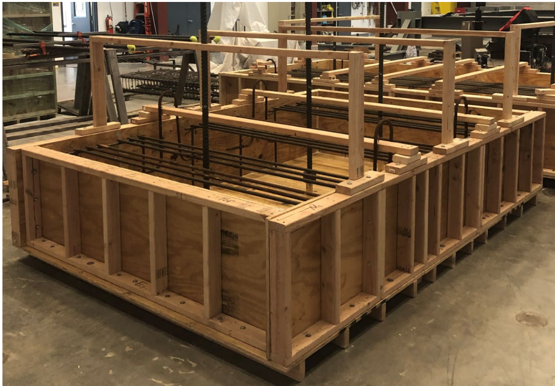
Figure 2.12 Slab specimen formwork
