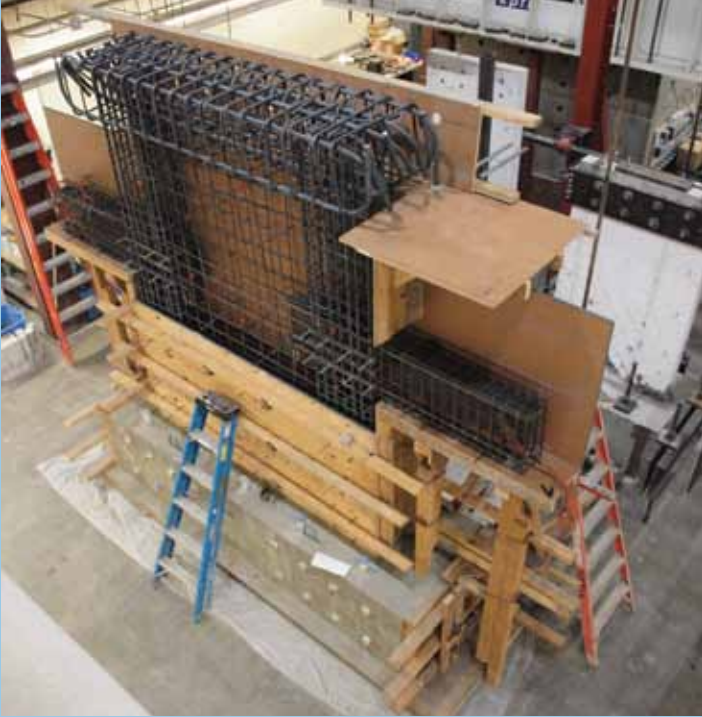
Steel sections, Composite Concrete Coupling Beams, UCLA
